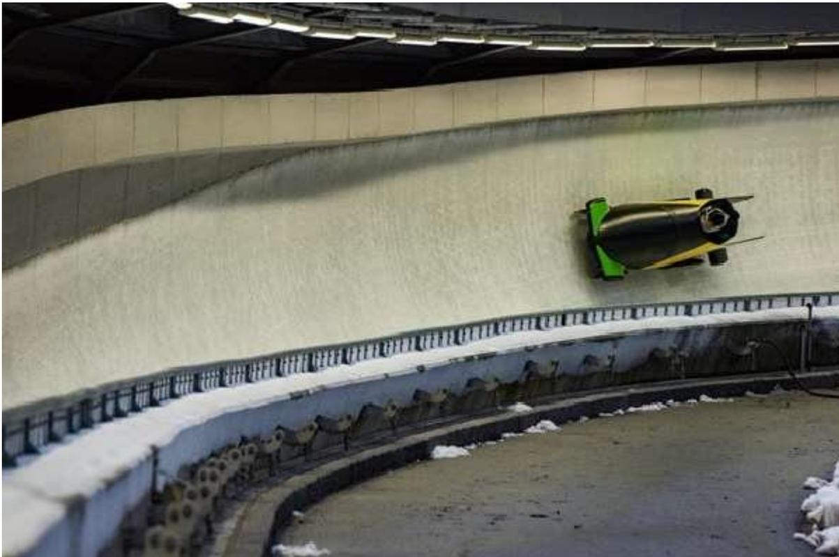
The track consists of narrow straightaway and curves which have deviation starting from smaller angles to 360 degree. These curves are banked almost 6 meters high above the ground where the racers can experience pressures that is four times the pressure of gravity.
