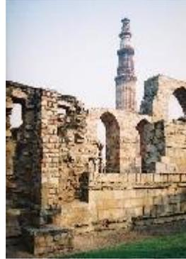
Qutub-Minar in red and buff sandstone is the highest tower in India. It has a diameter of 14.32m at the base and about 2.75m on the top with a height of 72.5m.
